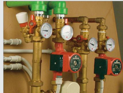
The Giacomini differential pressure valve R147N must be always installed downstream of the pump in between the supply and return pipes, the same versatility allows installation in both horizontal and vertical position respecting the flow direction marked (permanently) on the body itself of the valve.
